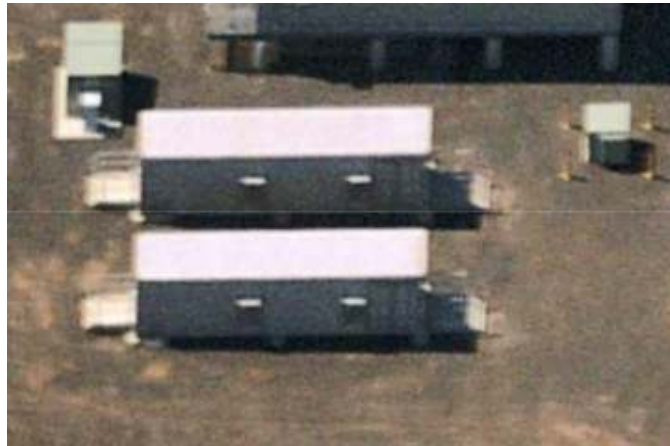
Image 6. 2 MWh Battery Installation at Deakin University Waurin Ponds
