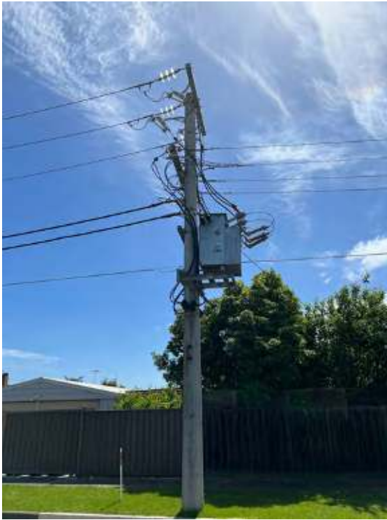
Image 13. Distribution Transformer
